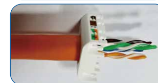
3.Placing the cable into the IDC cover.
